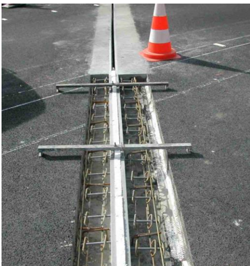
Installation lane by lane, to avoid traffic interruption
