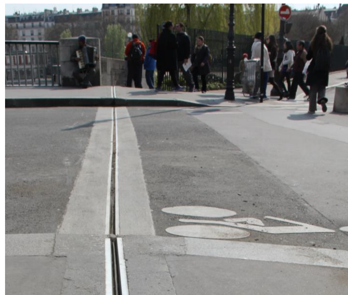
Saint-Louis Bridge, Paris (France)
