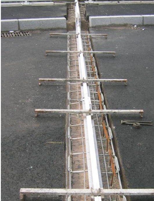
WRB joint during installation
