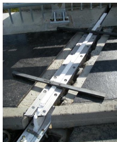
WOSd during installation: kerb treatment and footpath joint
