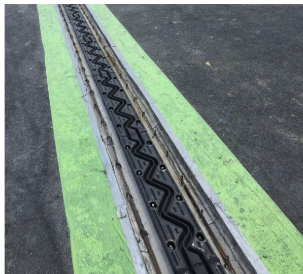
WM80 in the process of installation, Orly Airport (France)
