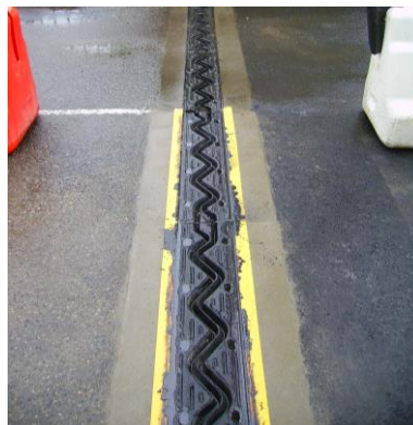
WM80 installed on Carennac bridge over the Dordogne river
