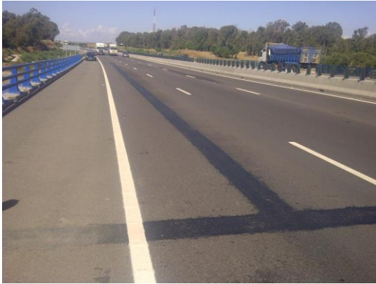
Longitudinal and transversal lines Oued Cherrat, Rabat-Casablanca Highway (Morocco)
