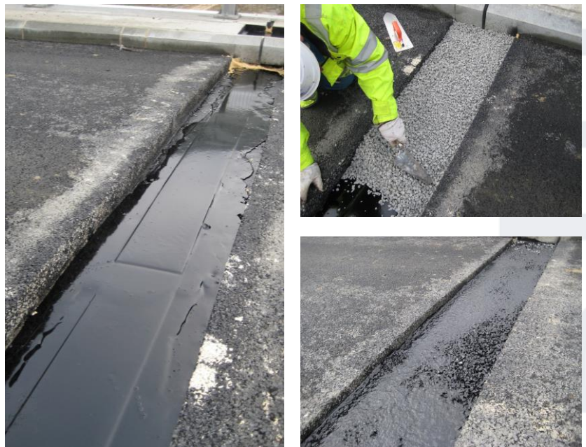
Viajoint® installation in successive phases
