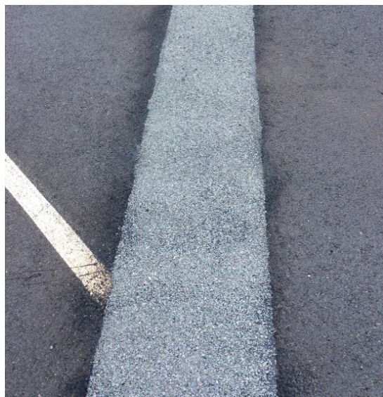
Different types of running surface finish ▲ with ▲ fine aggregates ▼ without ▼
