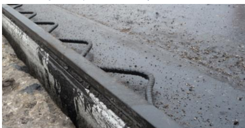
JEP welded to an orthotropic deck (Rouen, France)
