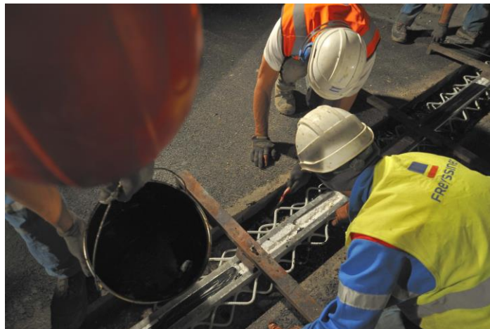
JEP joint installation on A1 Highway (France)
