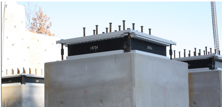
Bearings being installed
