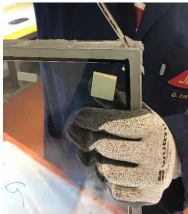
Figure 40: Pulling upwards the chisel
