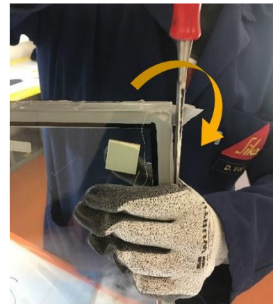
Figure 41: Pressing the chisel downwards
