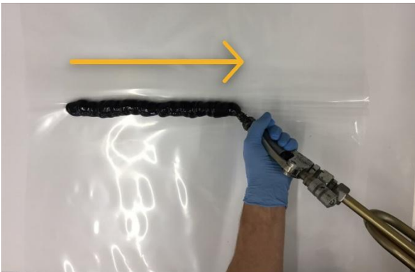
Figure 4: Apply the bead in the fold direction
